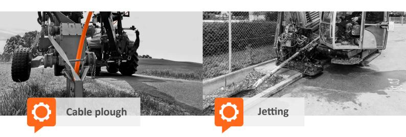
Cable ploughs plough a ditch parallel to the road. Ductwork or cable is then laid. This method is used in rural areas in particular and is considered a process-oriented method with a high degree of operational flexibility.
