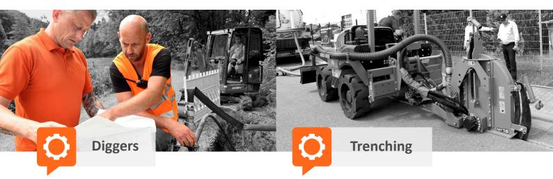
Diggers are a key part of conventional excavation. Trenches are dug and ductwork or cables are then installed. Due to the need to account for surface layers and soil types, only short stretches can be handled each day.
